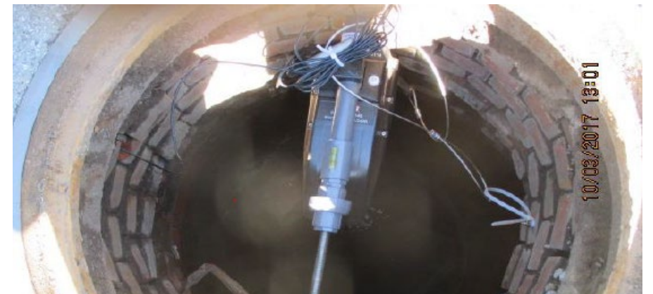
10 CSO meters were installed in 2017 within manholes to continuously monitor combined sewer overflows, a requirement of the NYSDEC.
