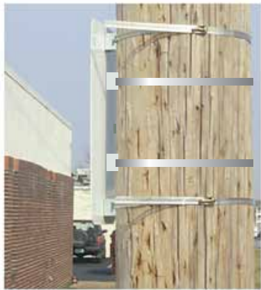
Band Bracket Detail Scale: N/A
