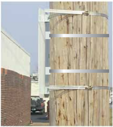
Band Bracket Detail Scale: N/A
