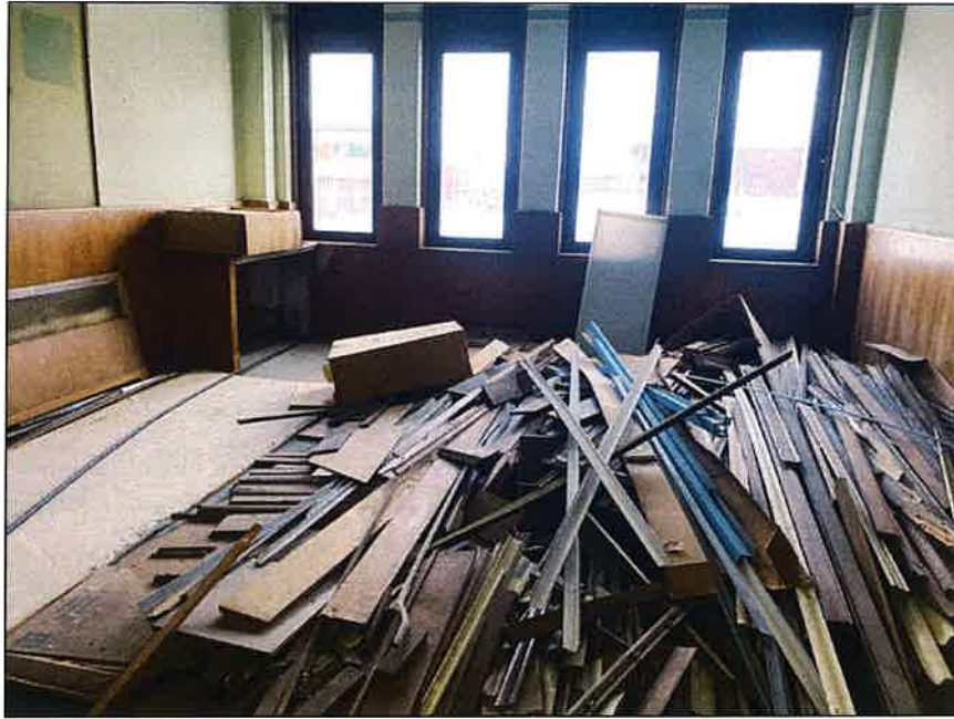
Photo 15: Building one; second floor
