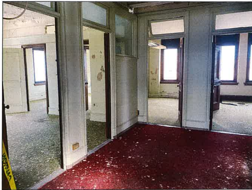
Photo 23: Building one; fourth floor
