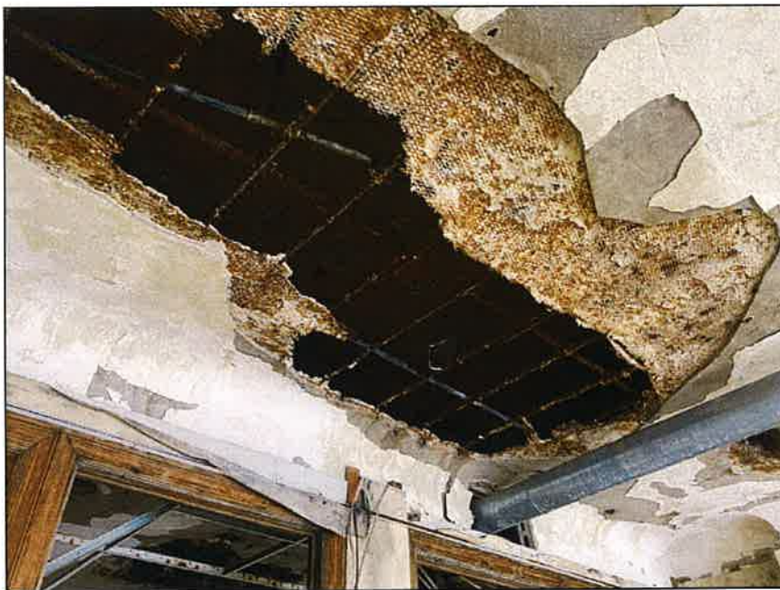
Photo 28: Building one; sixth floor ceiling
