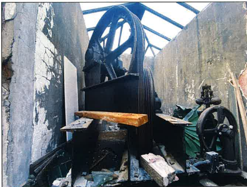
Photo 32: Building one; elevator equipment
