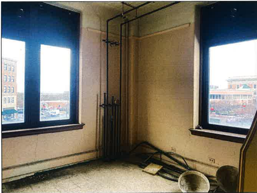
Photo 16: Building one; second floor
