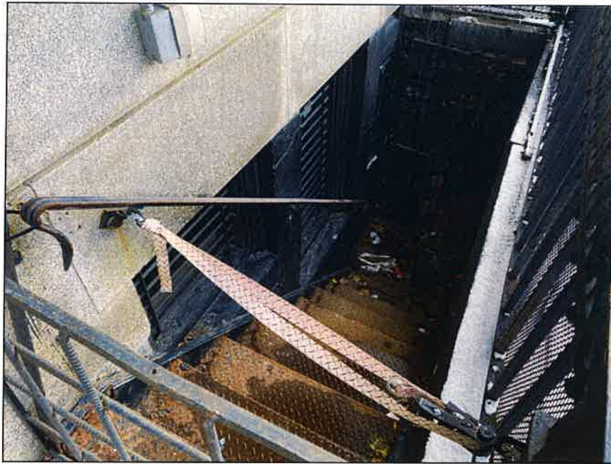
Photo 33: Building one; daylight basement
