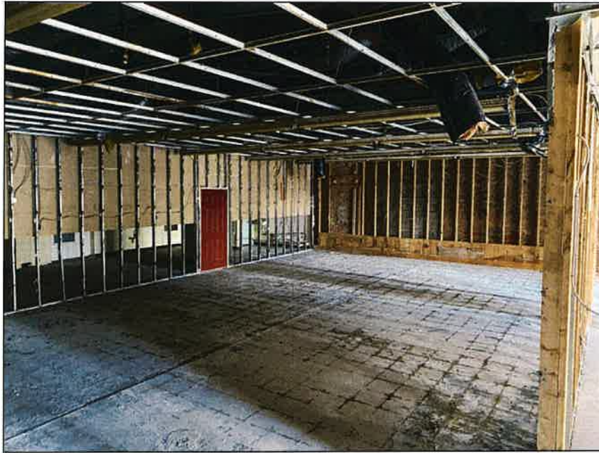
Photo 39: Building two; overview
