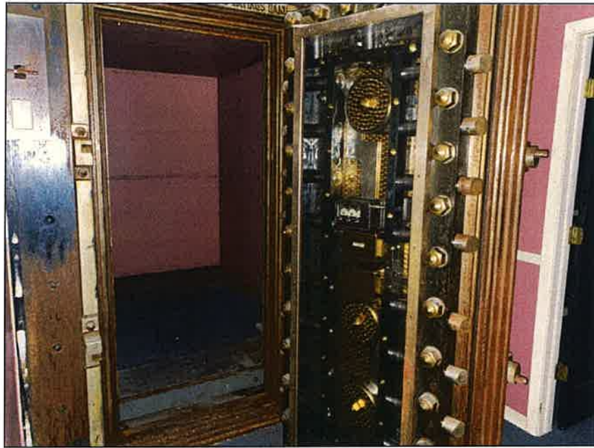
Photo 13: Building one; first floor former bank safe
