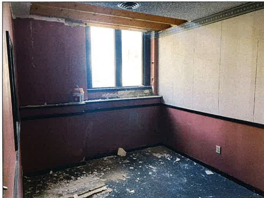
Photo 12: Building one; first floor
