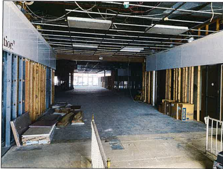
Photo 35: Building two; overview
