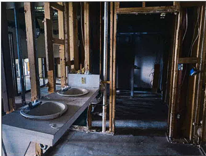
Photo 40: Building two; area of former bathroom
