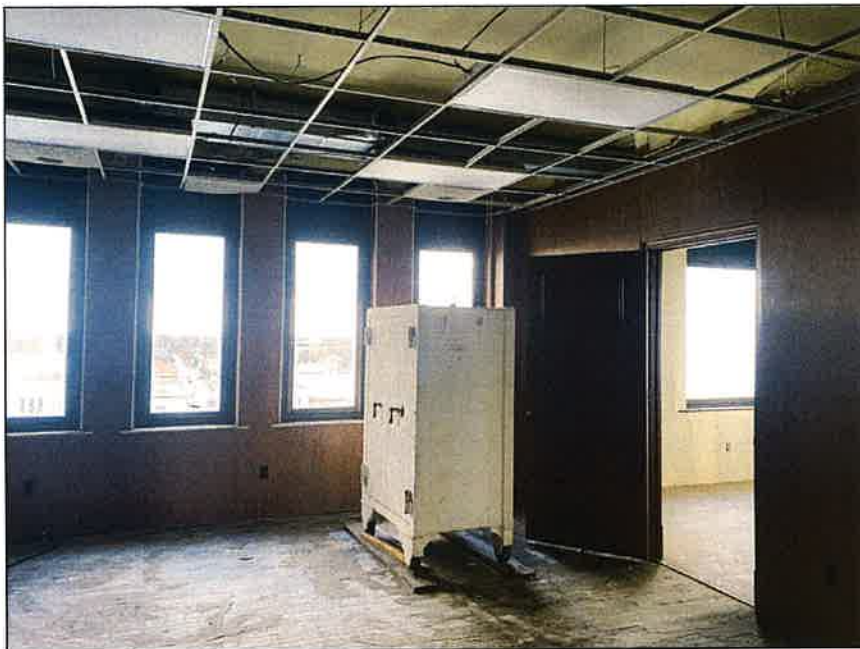
Photo 30: Building one; sixth floor
