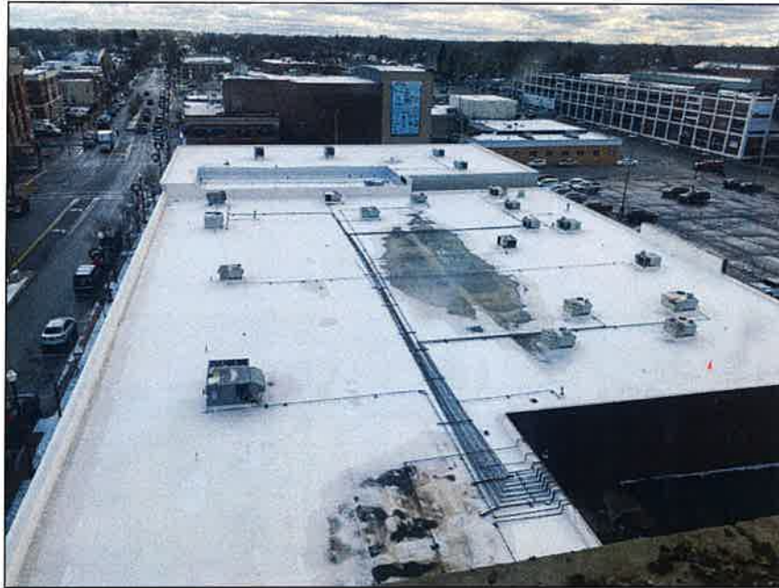
Photo 41: Building two; roof view
