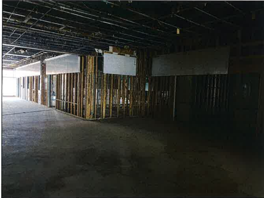
Photo 37: Building two; overview
