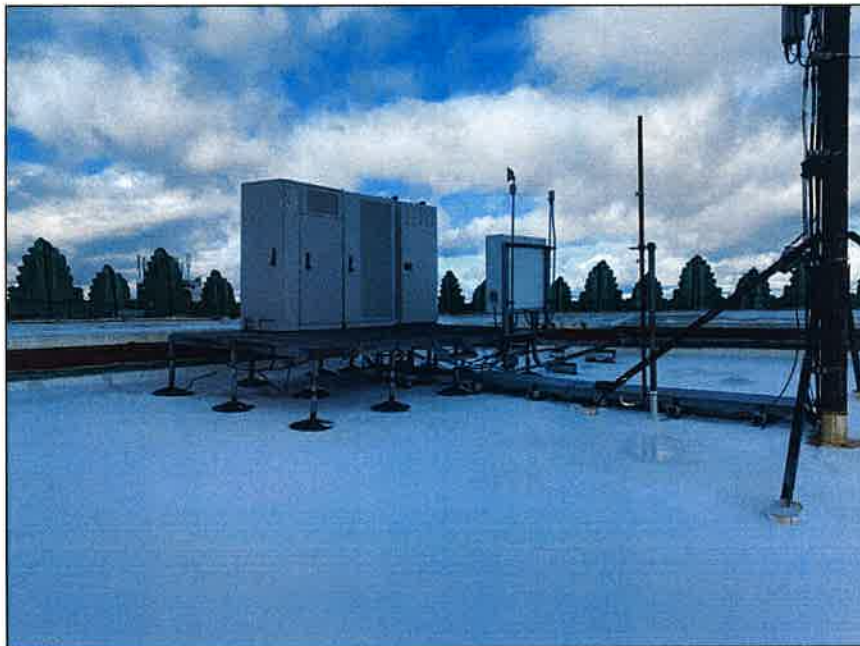
Photo 42: Building one; roof
