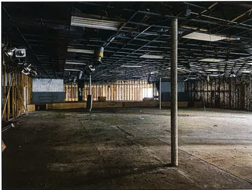
Photo 38: Building two; overview
