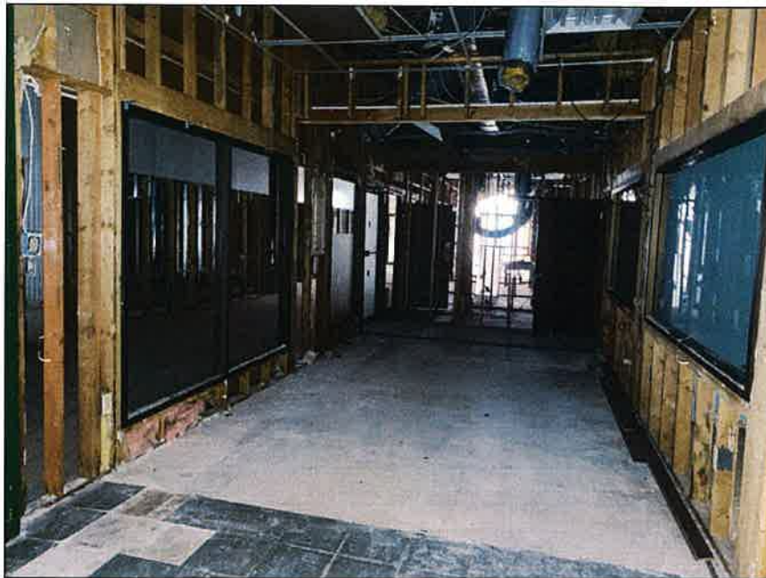
Photo 36: Building two; overview
