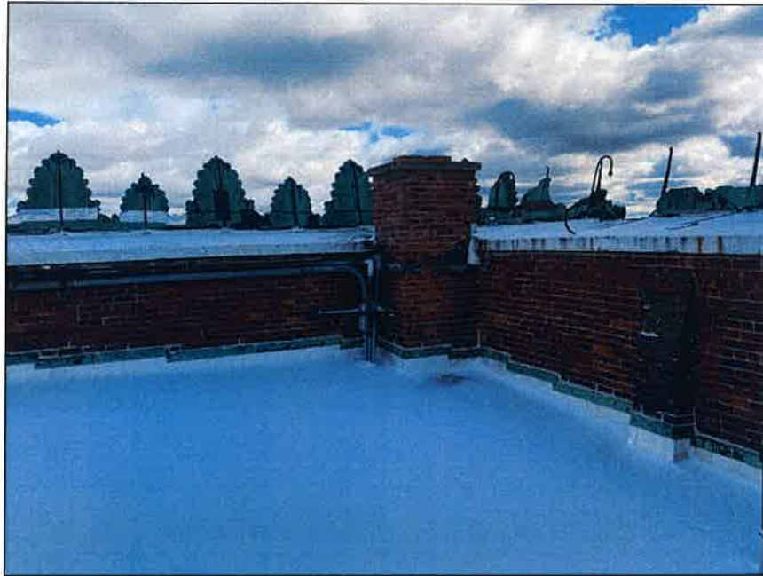
Photo 43: Building one; roof
