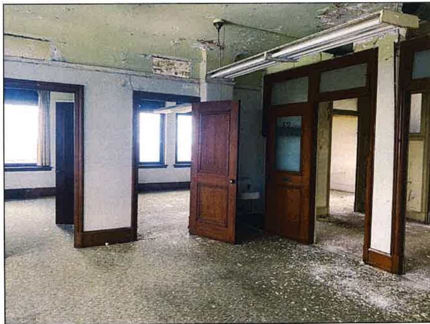
Photo 26: Building one; fifth floor
