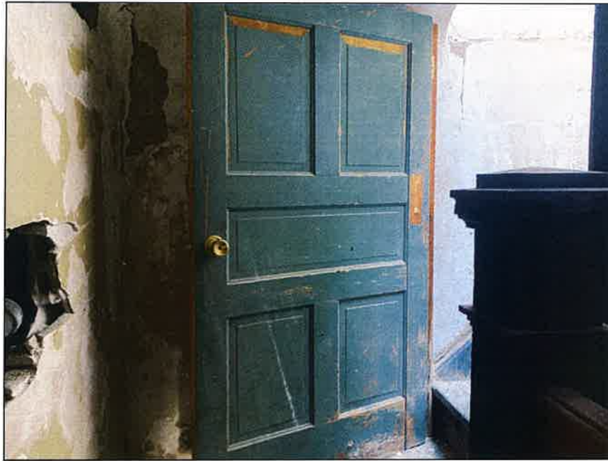
Photo 31: Building one; roof access
