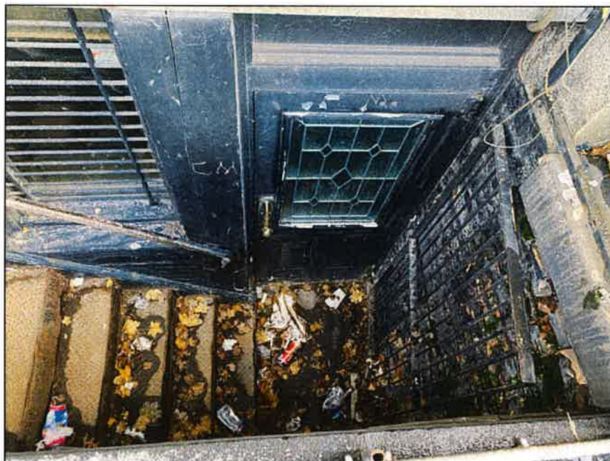
Photo 34: Building one; daylight basement
