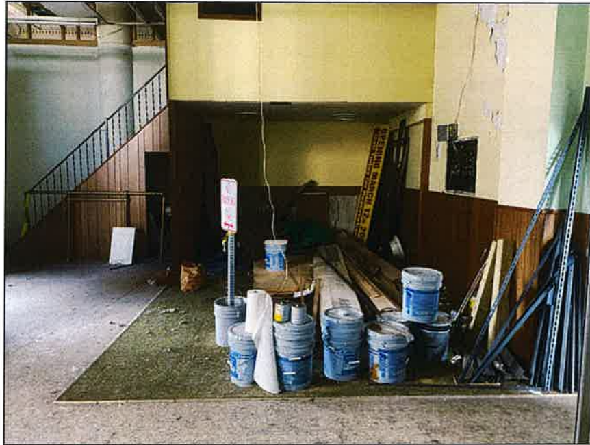
Photo 11: Building one; first floor maintenance paints
