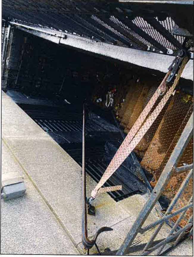
Photo 33: Building one; daylight basement
