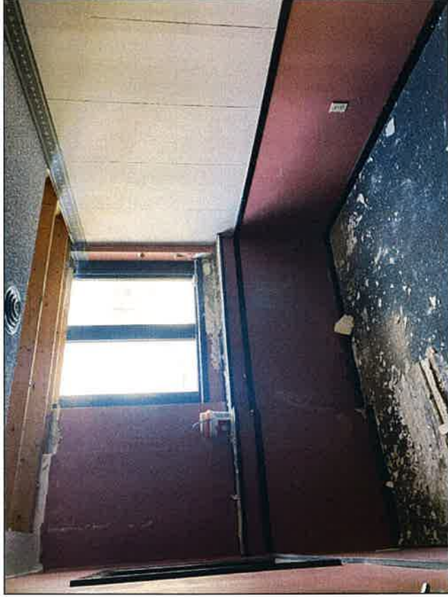
Photo 12: Building one; first floor
