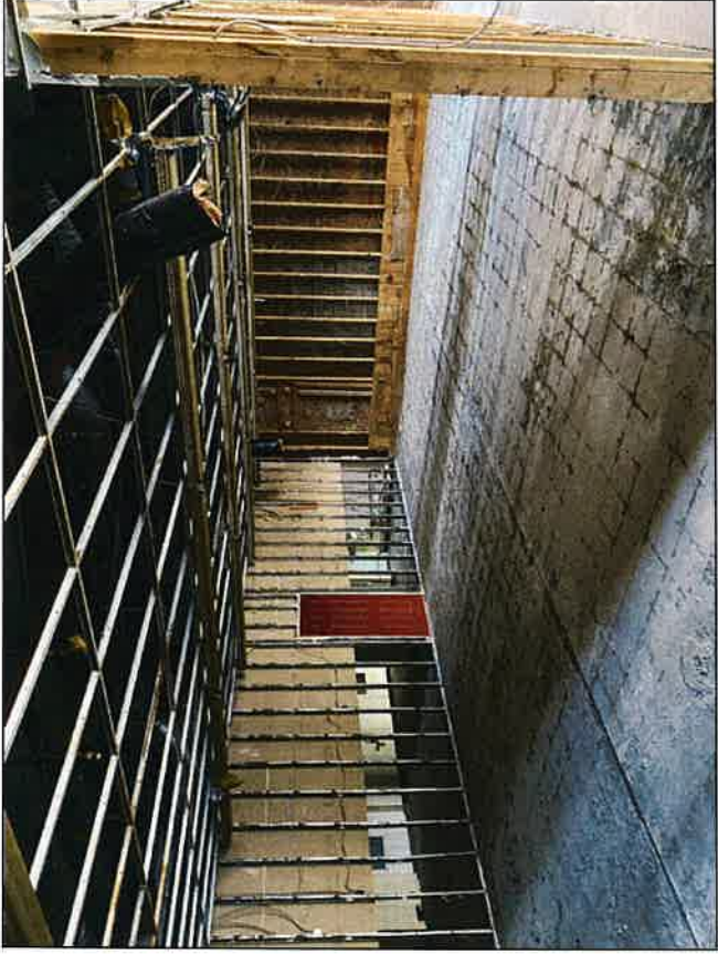
Photo 39: Building two; overview
