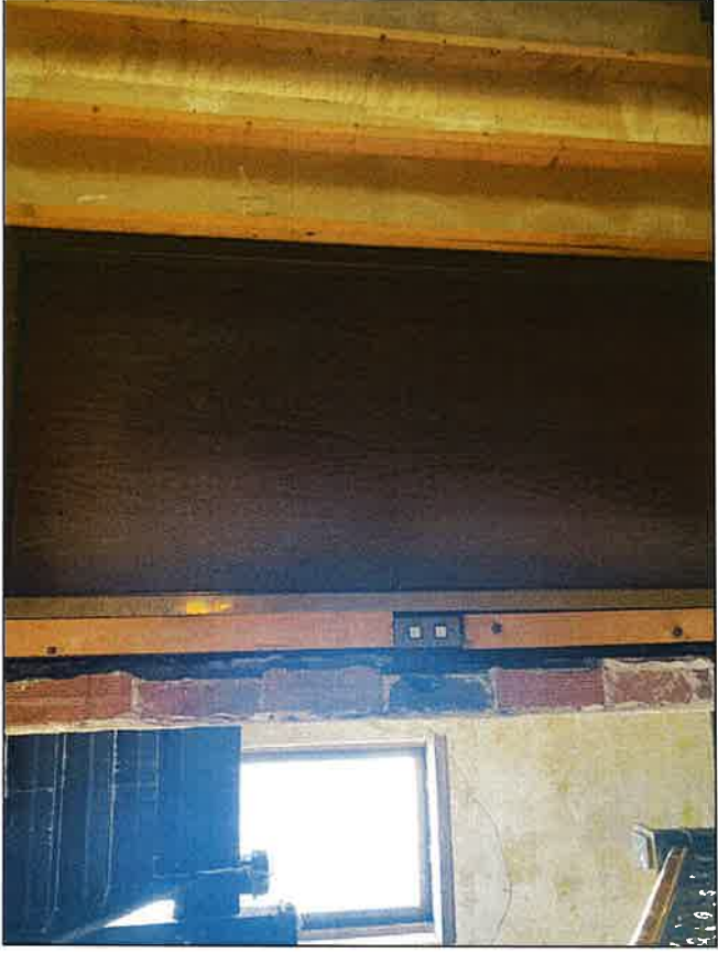
Photo 25: Building one; fourth floor elevator
