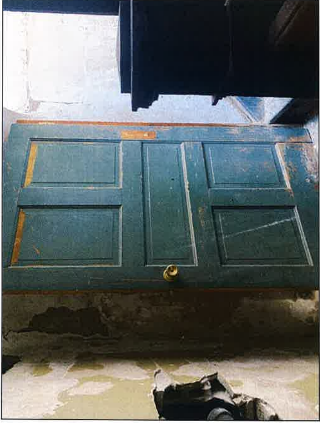
Photo 31: Building one; roof access
