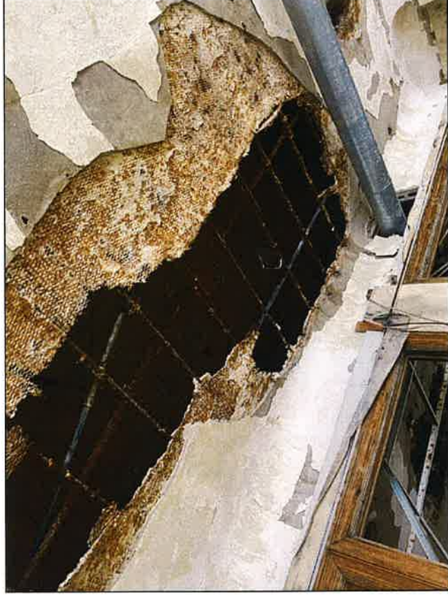
Photo 28: Building one; sixth floor ceiling
