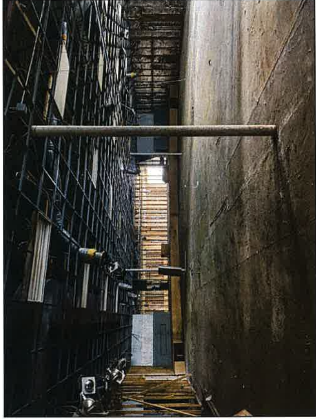
Photo 38: Building two; overview
