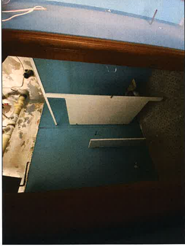
Photo 22: Building one; fourth floor bathroom
