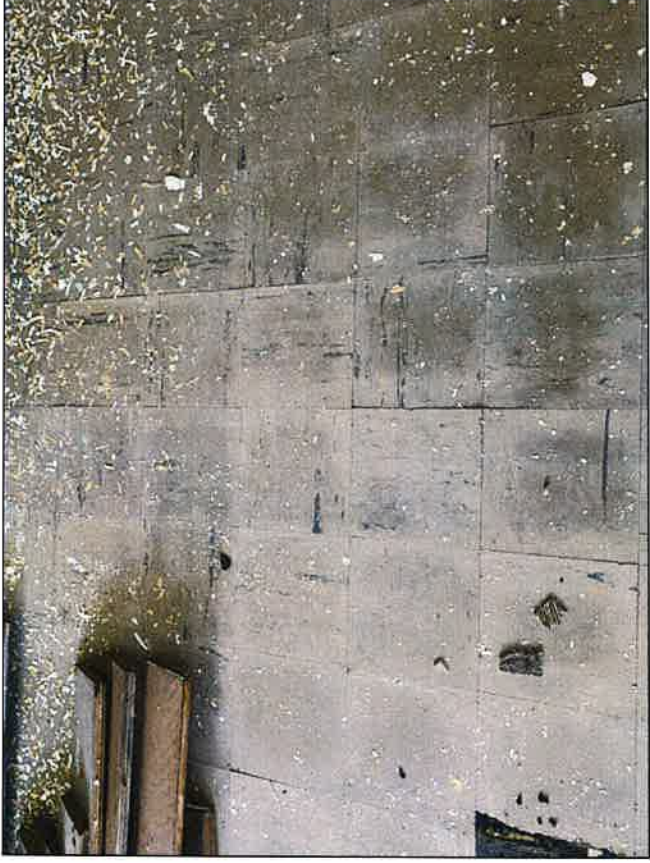
Photo 21: Building one; third floor 9"x9" floor tiles
