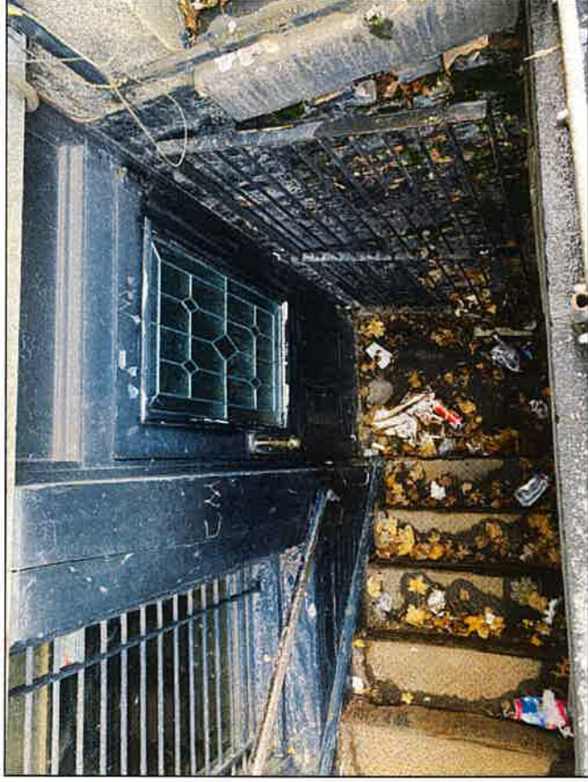
Photo 34: Building one; daylight basement
