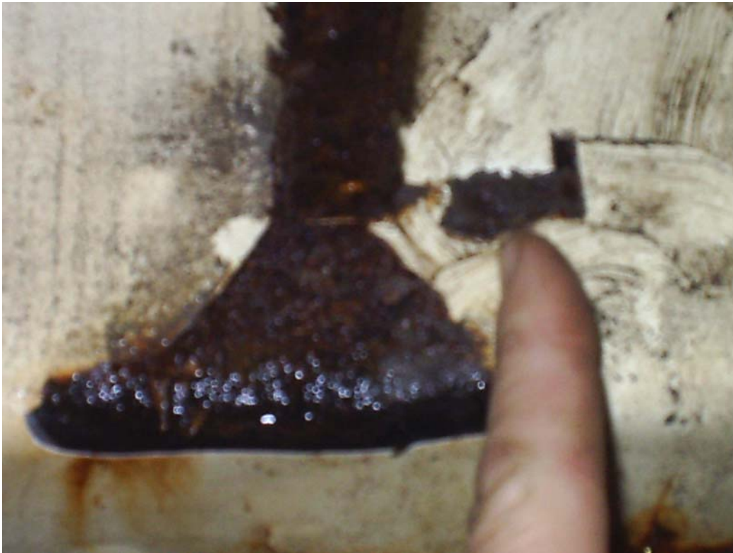
ADDITIONAL VIEW OF 1" X 1" FRAMING DETAIL WITH TAB DETERIORATION NEAR 100%.
