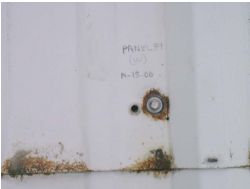
ADDITIONAL VIEW OF OLD SCREW HOLES DISCOVERED WITH NO INDICATION OF REPAIRS. HOLES ARE ALLOWING MOISTURE AND RAIN TO ENTER BUILDING AND SATURATE INSULATION.
