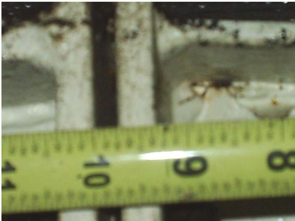
THE CAUSE OF DEFORMATION IS NOT CERTAIN. WE ARE RECOMMENDING CONNECTION BE SECURED WITH (4) NEW 2 1/2" X \phi 3/4" BOLTS.
