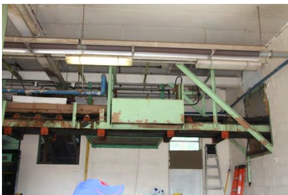
Figure 2-11. Sludge Conveyance System for Loading Trucks (above North Truck Bay)
