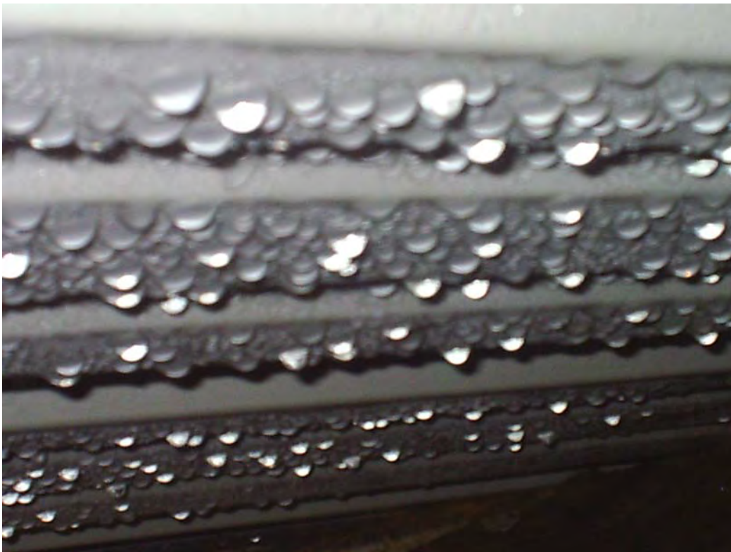
BOTTOM SIDE OF ROOF DECK, CONDITIONS FAVORABLE UNDER INSULATION (HEAVY CONDENSATION TYPICAL).
