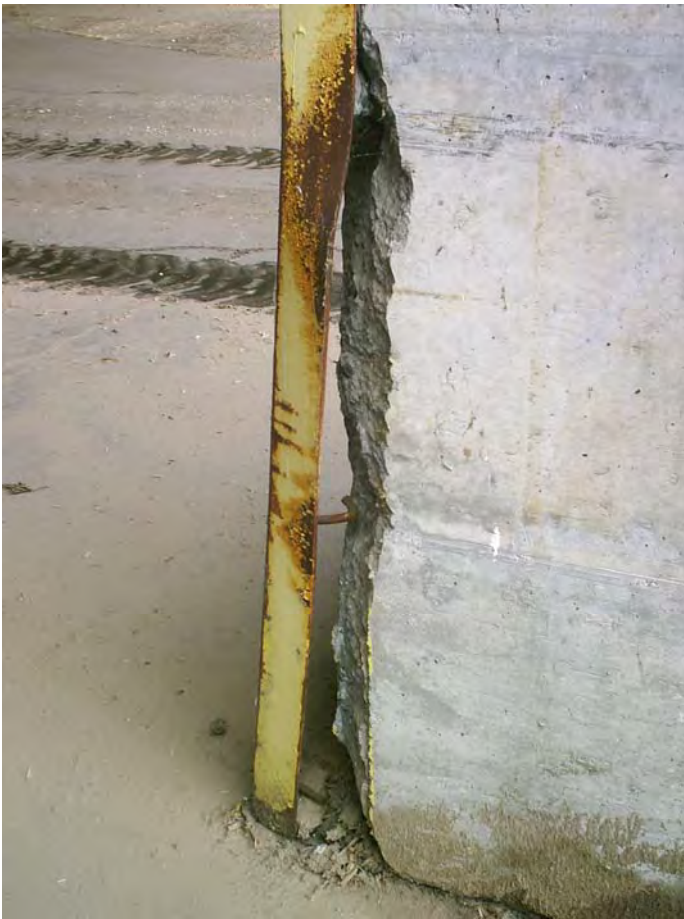
LEFT: OUTSIDE COVERED STORAGE AREA (G-17) COLUMN EXPERIENCING IMPACT DAMAGE FROM LOADER.
