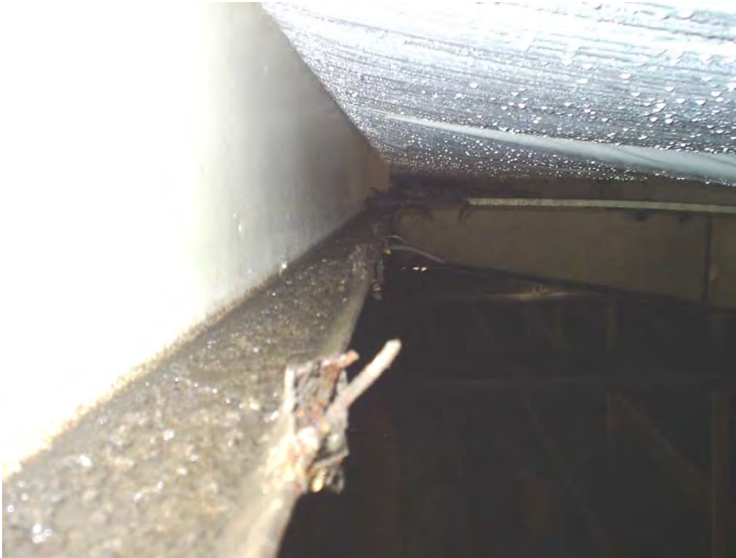
VIEW OF ROOF PURLIN CONDITIONS, INTERIOR OF BOTTOM FLANGE.
