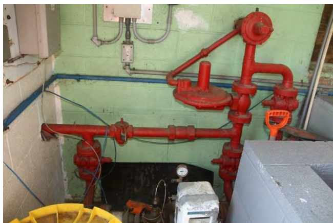
Figure 2-17. Natural Gas Service in Southeast Corner of Sludge Handling Room
