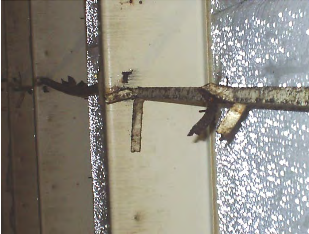
1" X 1" HORIZONTAL FRAMING ANGLES ARE ALSO EXPERIENCING MORE ADVANCED DETERIORATION WITH SEVERAL NEAR 100% SECTION LOSS.
