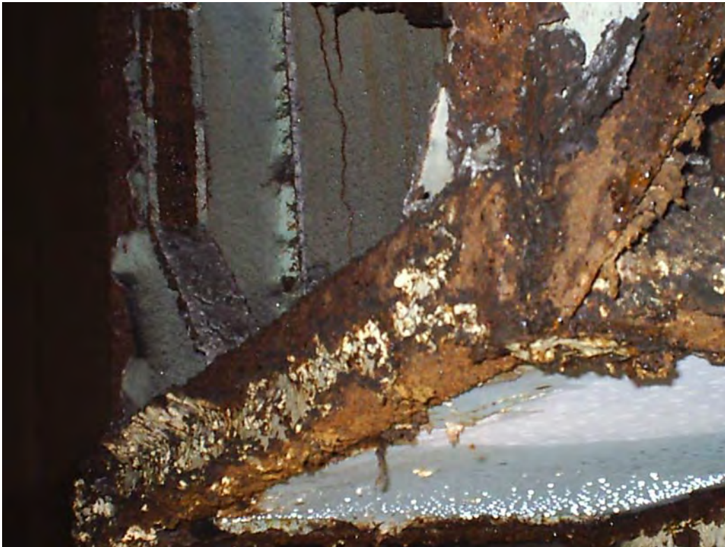
ADDITIONAL VIEW OF DETERIORATION ON FAN COMPONENTS. ALL (4) FANS SHOULD BE REMOVED IF NOT IN SERVICE.
