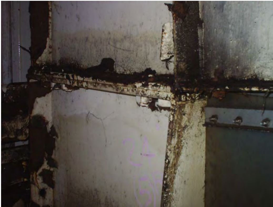
CORROSION AND SECTION LOSS PROGRESSING AT COLUMN GIRDER CONNECTION.
