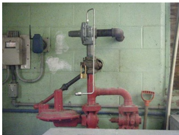
Figure 2-18. Natural Gas Service with Modified Blow-off Regulator
