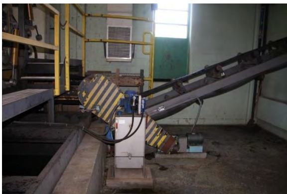
Figure 2-13. Conveyor from Belt Filter Press
