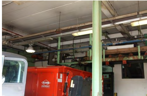
Figure 2-10. Sludge Conveyance System for Loading Trucks (above South Truck Bay)
