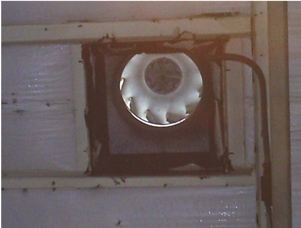
ROOF FANS IN MIXING AREA DEVELOPING ADVANCING COATING DETERIORATION AND EDGE CORROSION.
