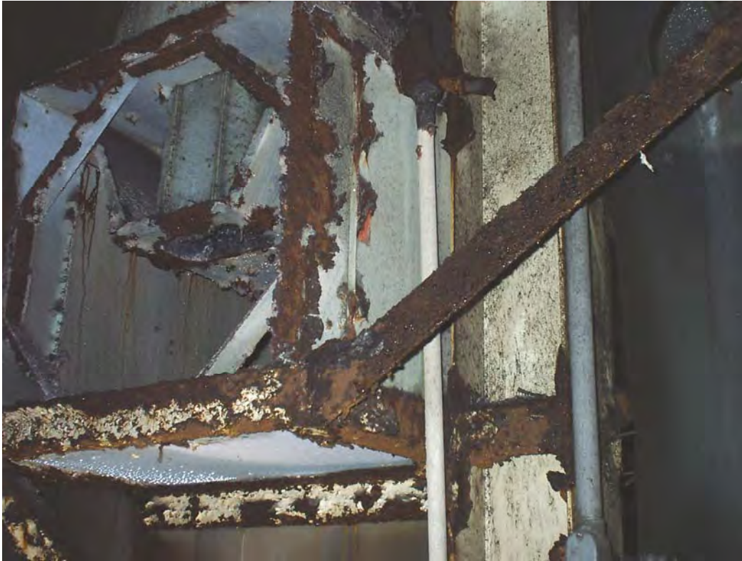
OLD FANS AT MIXING TO COMPOST TRANSITION ARE EXPERIENCING SIGNIFICANT SECTION LOSS ON SUPPORT DETAILS.
