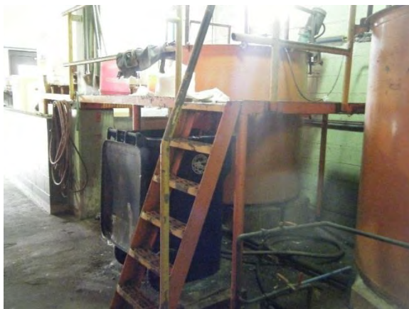
Figure 2-15. Polymer Tanks on South Wall of Sludge Handling Room
