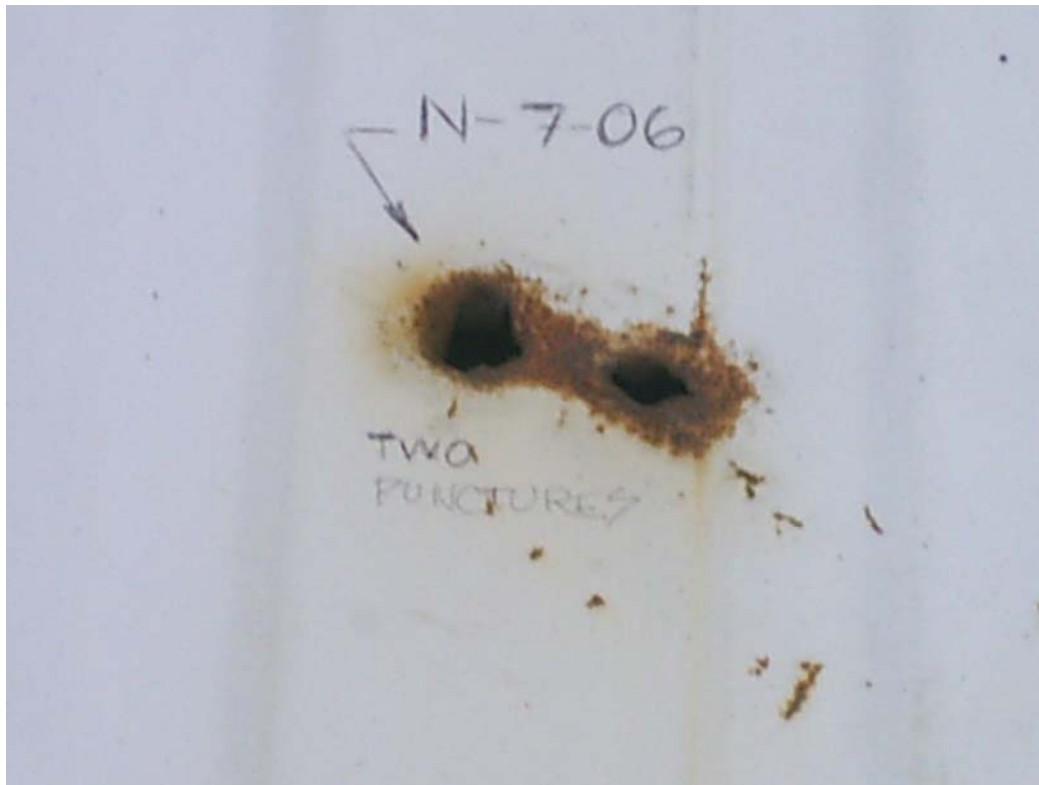
DURING OUR SURVEY, NUMEROUS PUNCTURES AND HOLES WERE NOTED (VIEW OF N-7-06) AT PANEL 42-EAST.
