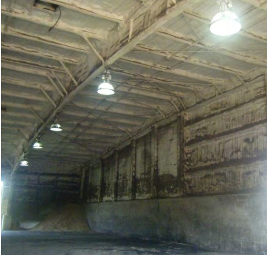
Figure 2-2. Compost Facility - Roof Decking with Stayflex Coating System
