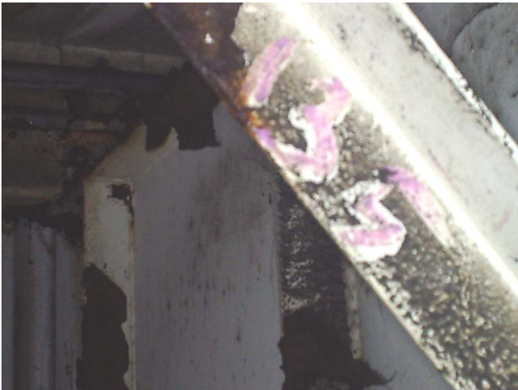
PHOTOGRAPH OF ULTRASONIC TESTING 2" X 2" FRAMING ANGLES.
