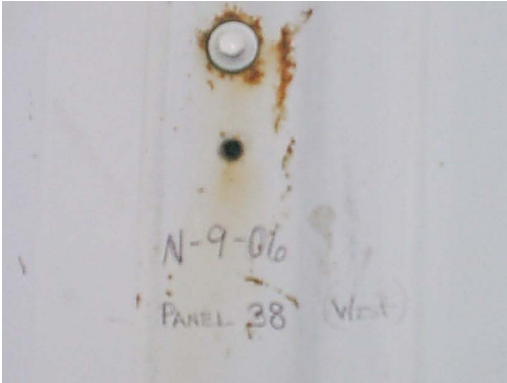
PHOTOGRAPH OF N-9-06, OLD SCREW HOLE FROM DRILL MISS NEVER REPAIRED.
