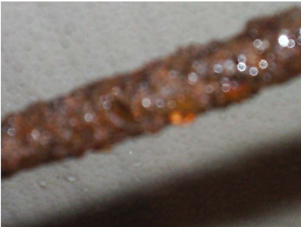
ZOOM VIEW OF X-BRACE (SWAY) WITH 32% SECTION LOSS. PROTECTIVE COATINGS RECOMMENDED IN THE REASONABLE NEAR FUTURE.
