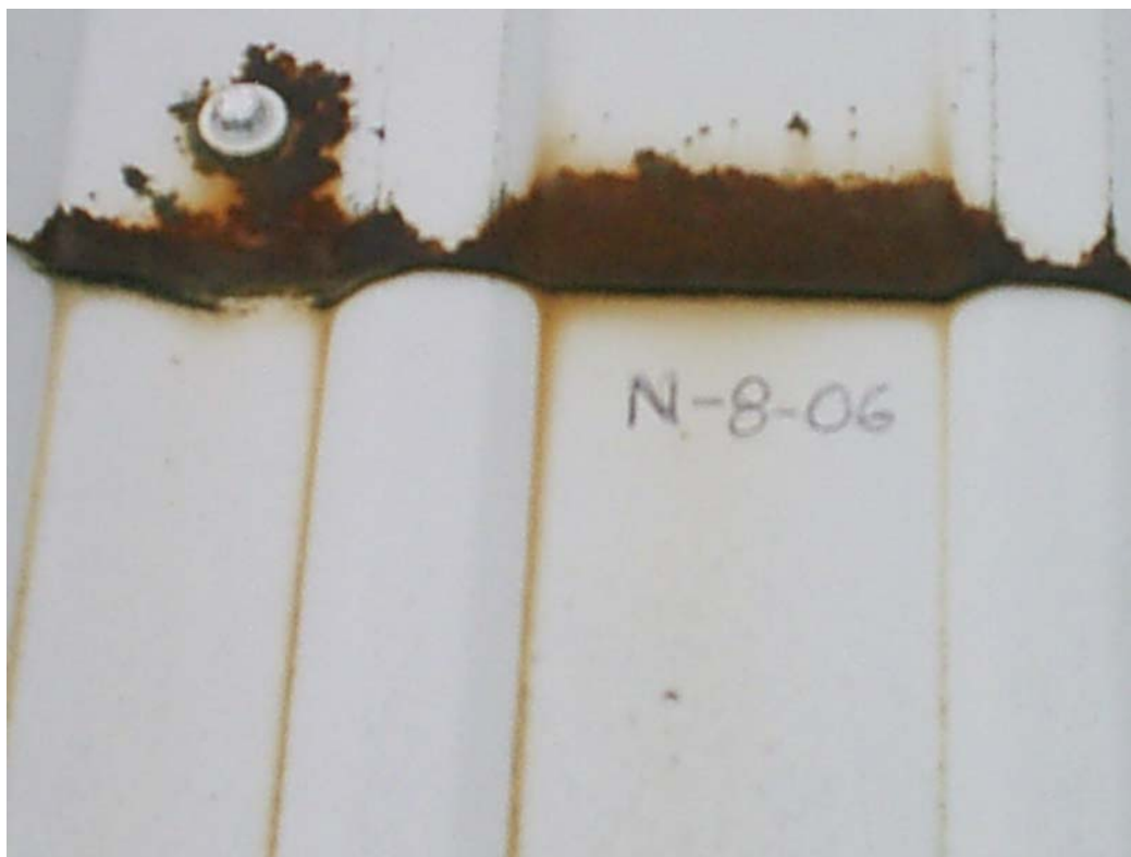
ADDITIONAL VIEW OF ADVANCING COATING DETERIORATION, ALL AREAS.
