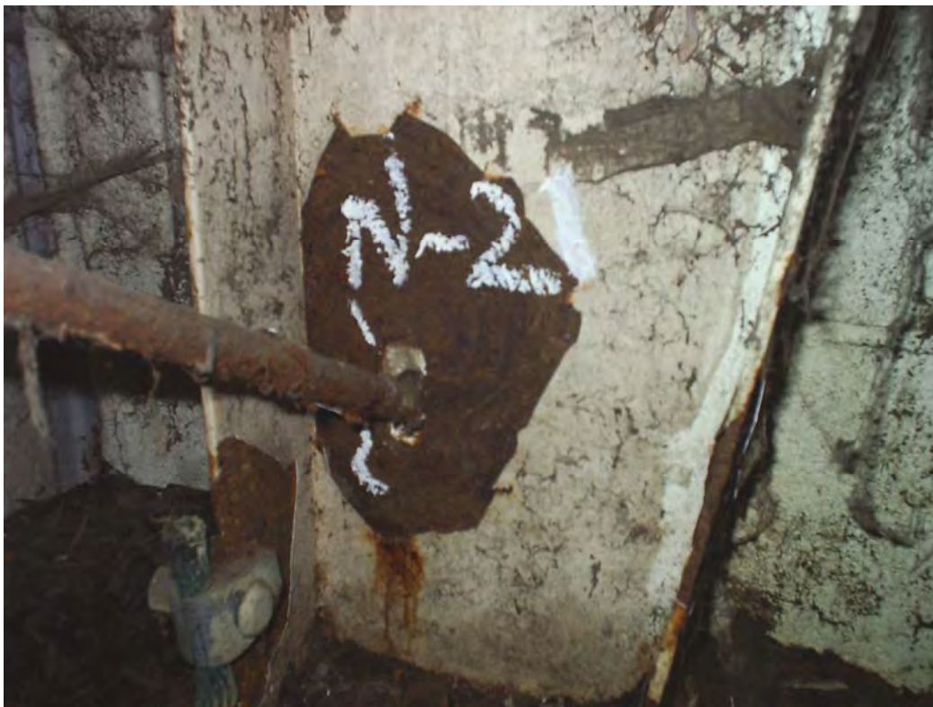
TWO FRACTURES WERE DISCOVERED IN WEB AT X-BRACING IN MIXING AREA (A-15). FRACTURES WERE 1/4" AND 3/4" LONG.
