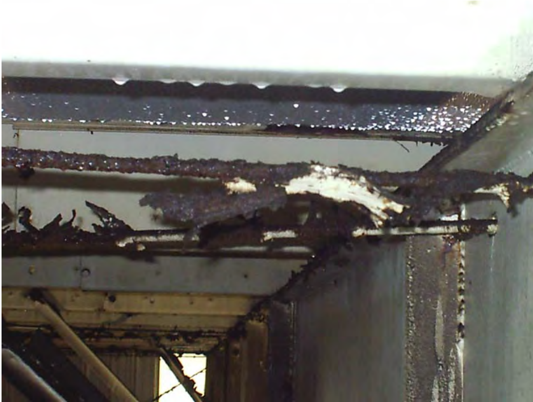
PHOTOGRAPH OF ROOF X-BRACING WITH NOTABLE LOSS OF SECTION.
