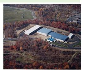
WeCare operates and maintains a state-of-the-art composting facility, utilizing the in-vessel BDP ICS composting technology, processing 100 wet tons per day of biosolids and 80 tons per day of wood/yard trimmings. WeCare sells all finished compost under the WeCare Compost® label to soil manufacturers, landscapers, and various turf-grass applications.
