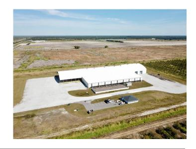
Denali Water owns and operates nuTerra SE FL Organics aerated static pile (ASP) composting facility located Indian River County, in Fellsmere, Florida. The facility manages merchant biosolids and yardwaste, which are delivered to the facility 6 days per week.
