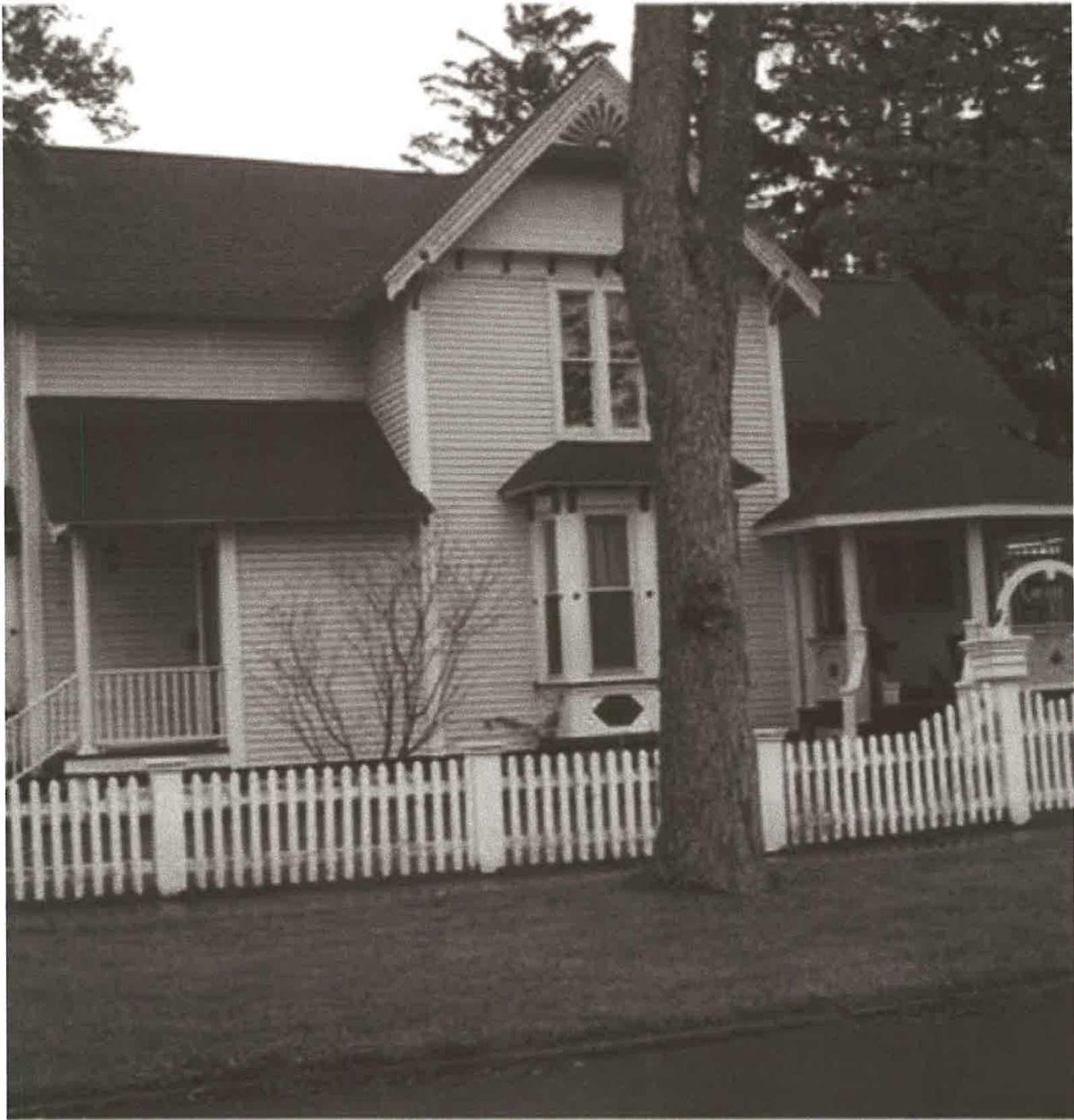
Vine Street side existing
