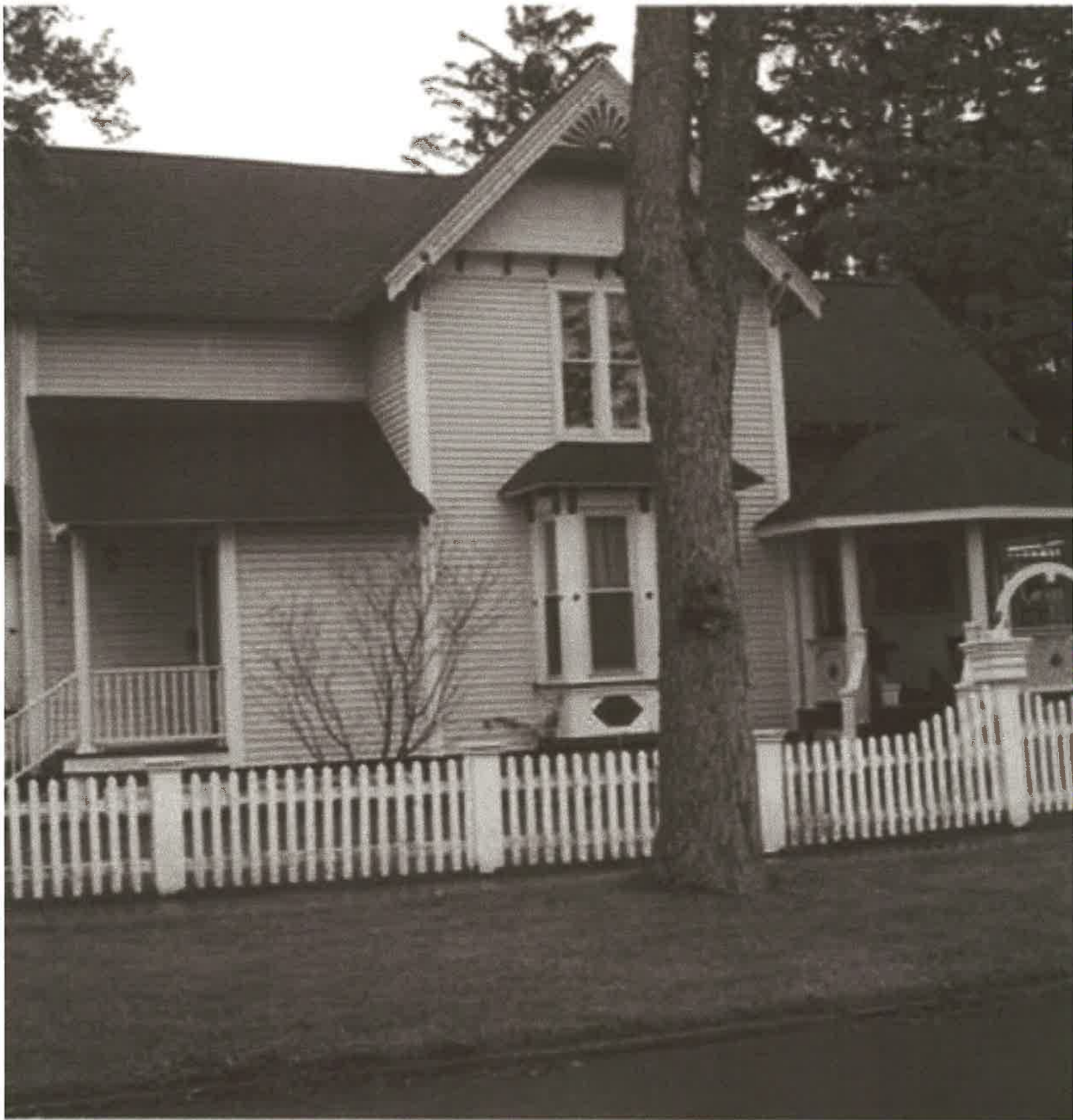
Vine Street side existing
