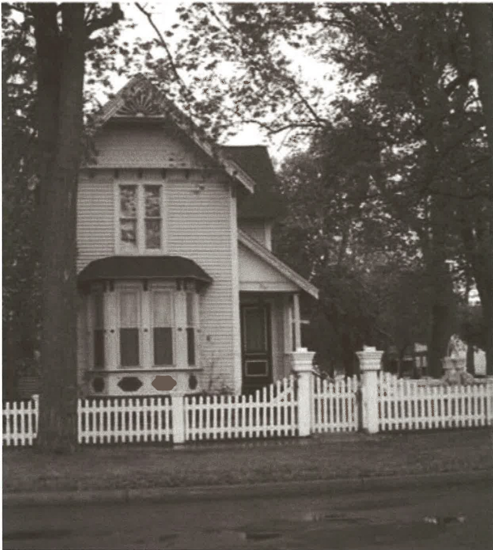
East arc side existing
