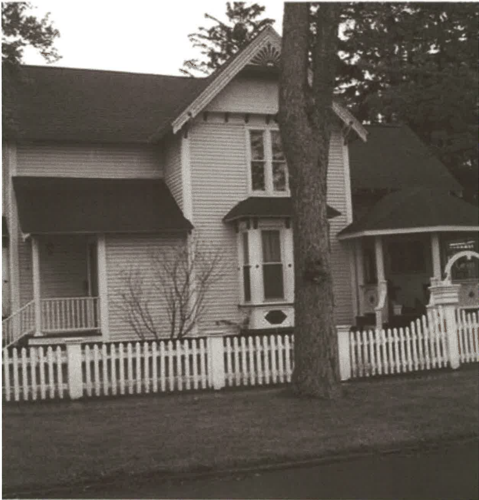
Vine Street side existing
