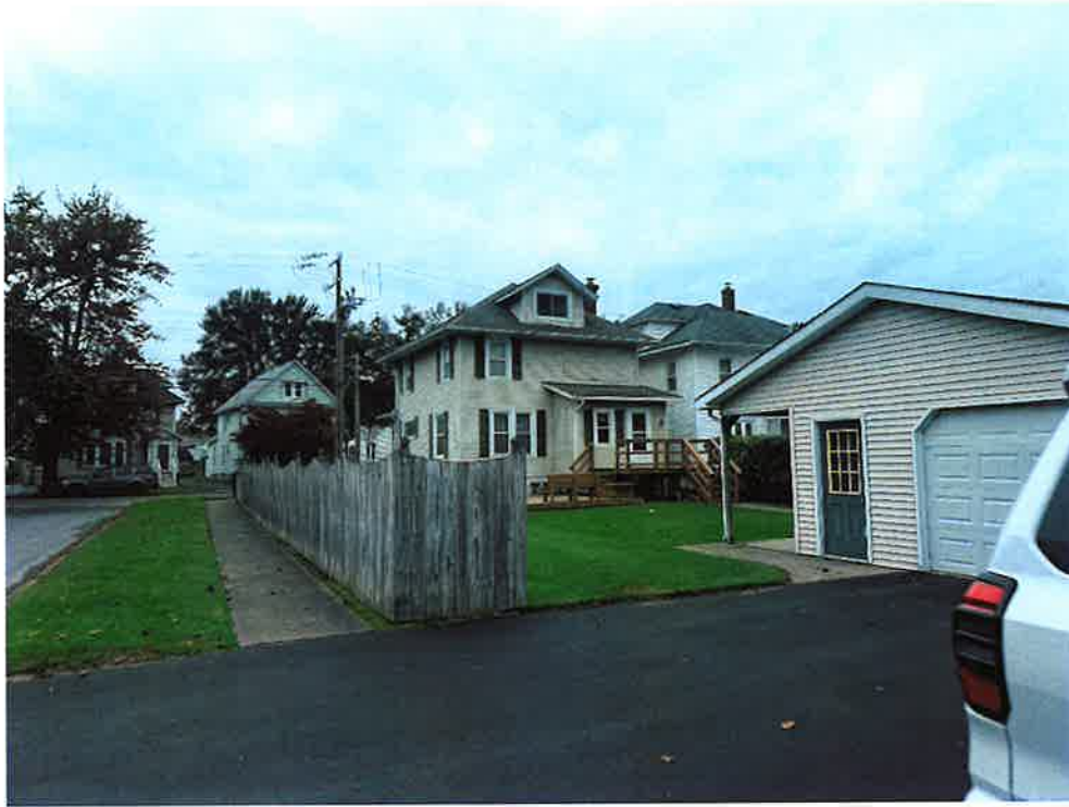
68 Harrison Ave, Lockport, NY – Approx. 2 blocks away
